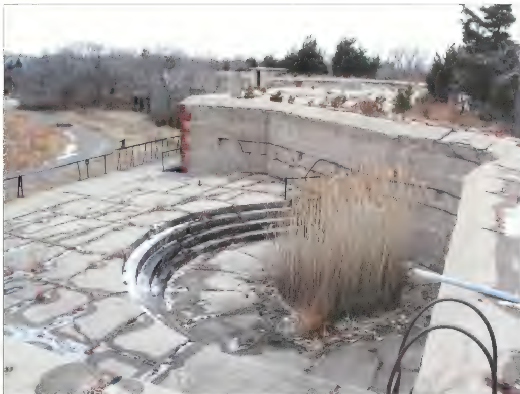
Figure 5.46. View of phragmites in gun well #6, Nine Gun Battery. Phragmites should be cut just after tasseling and the remaining stems should be treated with a hand-swiped application of a glyphosate herbicide (Olmsted Center, January 2009).
